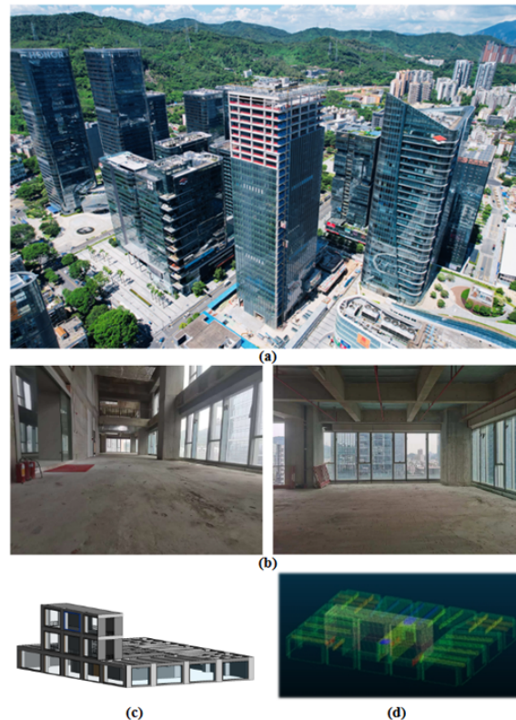
Figure 18. Experimental site. (a) Actual project; (b) Photos of the experimental site; (c) BIM of the experimental site; (d) Point cloud model based on BIM. BIM: building information model.
