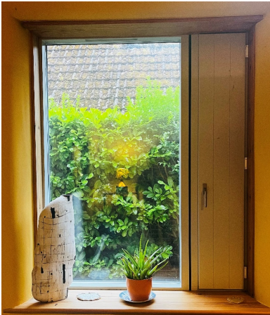
Figure 3. Internal view of insulated vent panel providing secure ventilation in the home office (image by the architect).
